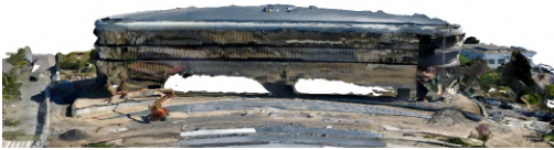
Figure 7: Large holes in the building as an example of texture failure after poor image alignment in Aerial Model.
